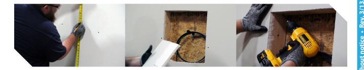
If the preference is for the enclosure to be installed first then drywall around the enclosure by measuring the distance from the floor and cutting appropriate sized drywall sheets then use the included Multilink spacers between the enclosure mounting flange and the stud to offset the enclosure from the stud to accommodate drywall thickness.
